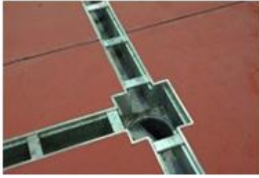
Lined channel detail
