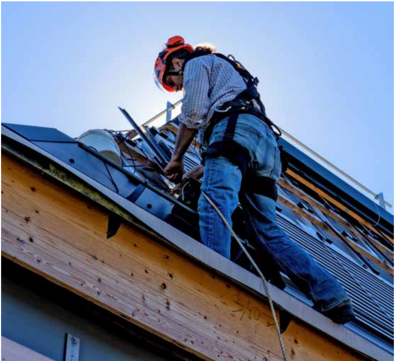
The sloped metal roof is waterproofed by Sarnafil® TG66-15 membrane system including 2 layers of mineral wool thermal insulation.
