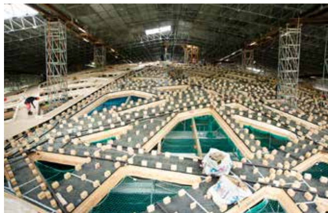
Roof structure of the elephant park
