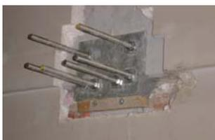
Fig. 7: Base plate on prestressing side in the roof space
