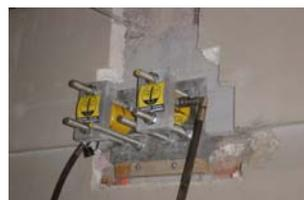
Fig. 9: Hydraulic presses in the roof space pulling the threaded rods outwards
