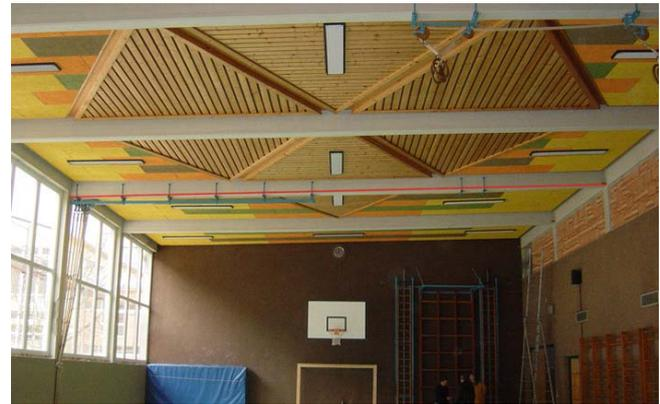
Fig. 2: Interior view: 5 reinforced concrete trusses to be strengthened
