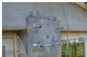
Fig. 8: Base plate on fixed side outside
