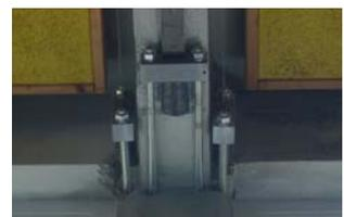
Fig. 10: Prestressed CFRP plates before bonding
