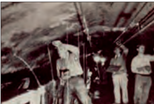
Impermeabilisation of Lötschberg (Switzerland) railway tunnel
