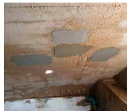
Pulling tests on repair mortars.
