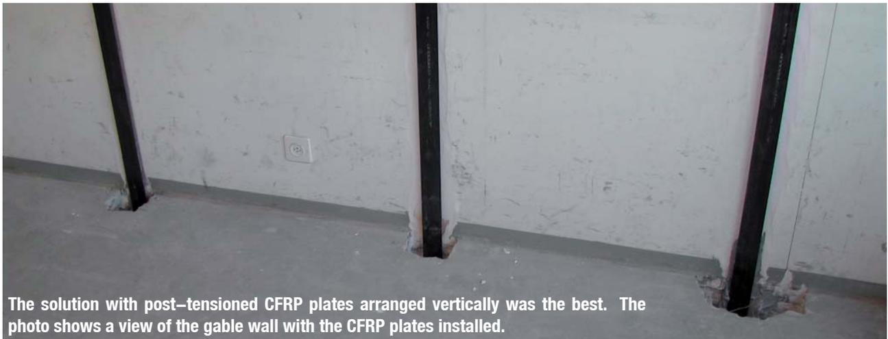
The solution with post-tensioned CFRP plates arranged vertically was the best. The photo shows a view of the gable wall with the CFRP plates installed.
