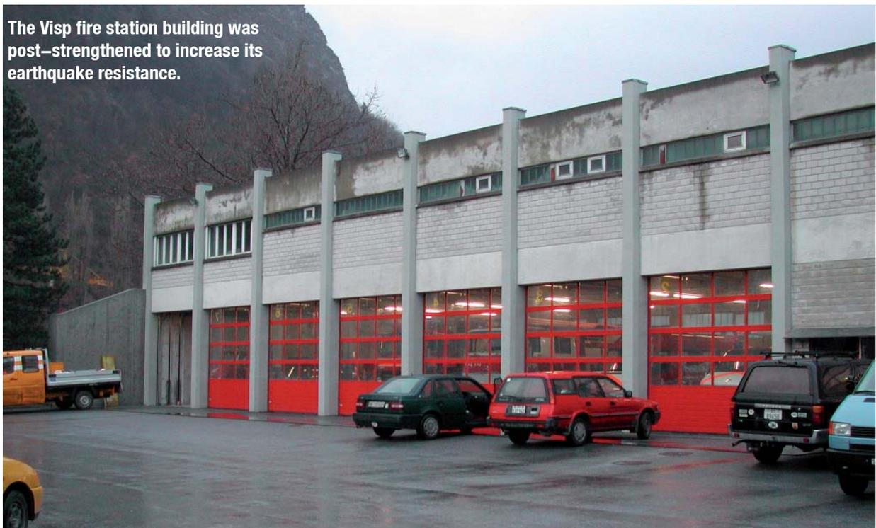
Finally the most efficient and cost effective method selected was an innovative solution with post-tensioned CFRP plates arranged vertically. This vertical post-tensioning of the masonry has increased the load resistance to horizontal forces so much that the stress from earthquakes can now be dissipated entirely through the masonry in accordance with the latest European Standards. This also secures and prevents the infill panels collapsing out of the frame.
