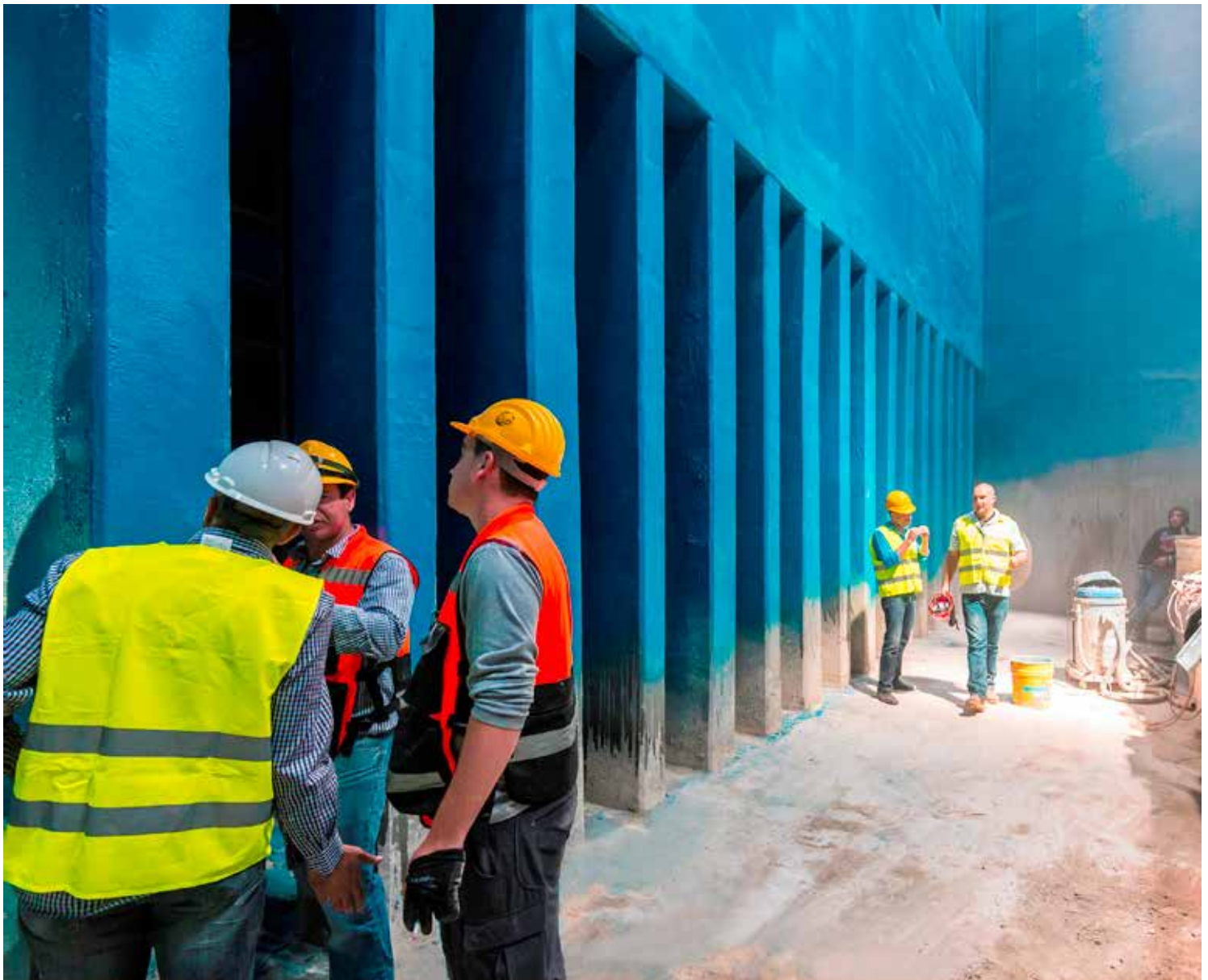
After the appropriate professional surface preparation by high-pressure water jetting, all surfaces are leveled with Sikagard®-720 EpoCem, followed by an epoxy primer, SikaFloor®-156. Every inch of the surfaces, covering 20,000 m 2 , spray Polyurea, Sikalastic®-841 ST.
