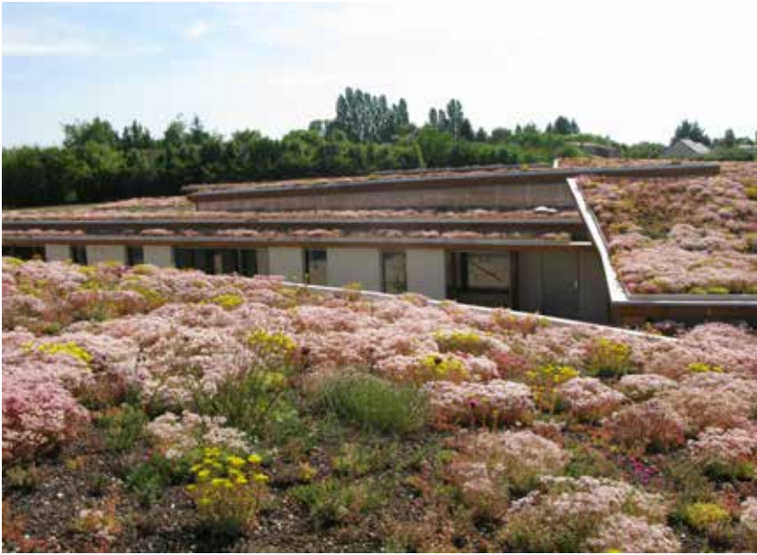
Saint Doulchard Medical Center, Cher, France Project year: 2010
