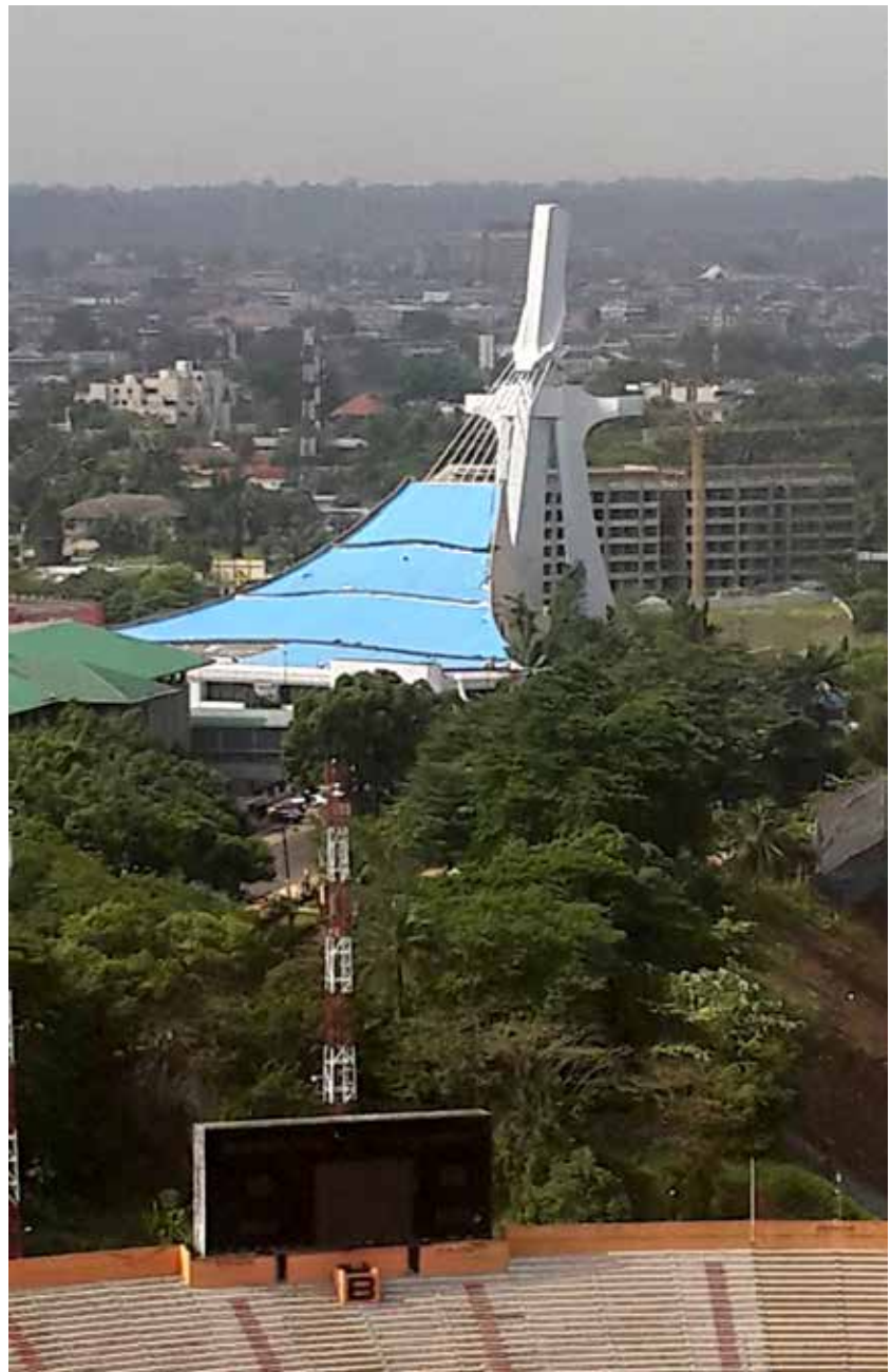
The roof of the Abidjan cathedral needed major refurbishment and Sika was chosen by the government to undertake this.
