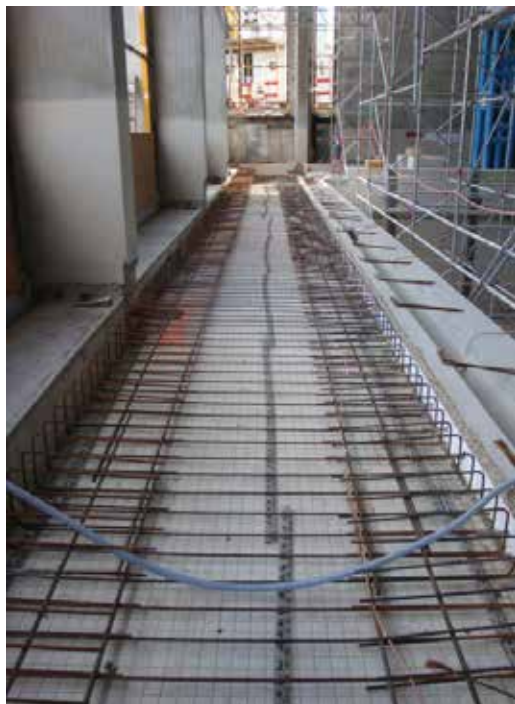
During works of refurbishment.
