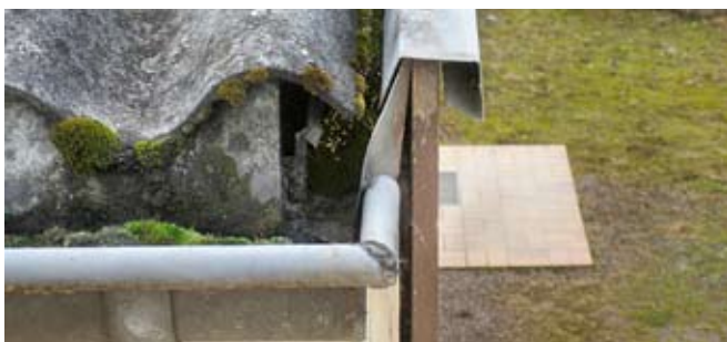
The old roof before refurbishment
