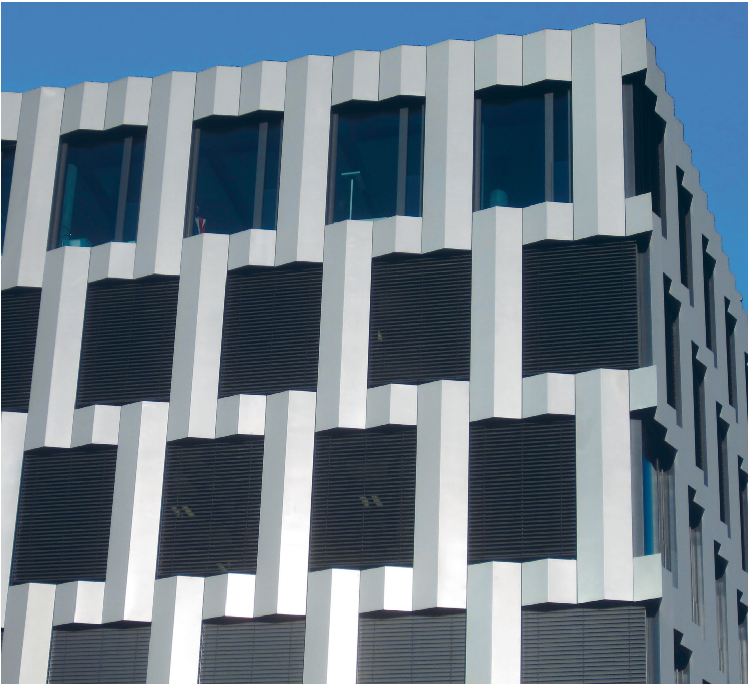
Office Building Zurich West, Zurich, 2013 Facade Yuanda Europe
