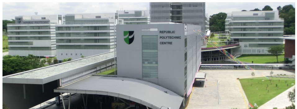
Republic Polytechnic Center, Singapore, 2006 Architects Fumihiko Maki, DP Architects; Sealed with Sikasil® WS-605 S, after >10 years no signs of streaking effect
