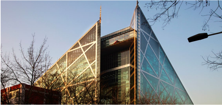
Park View Green Plaza, Beijing, 2010 Consultant ARUP Hong Kong; Facade Beijing Jianli (CN)
