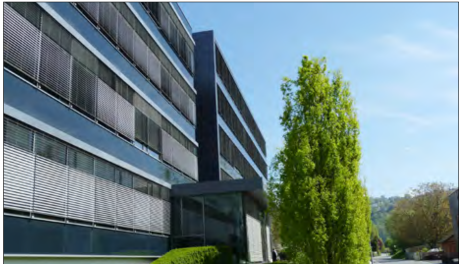
Fig. 2: Front view of the Meusburger Building in Wolfurt (Austria)
