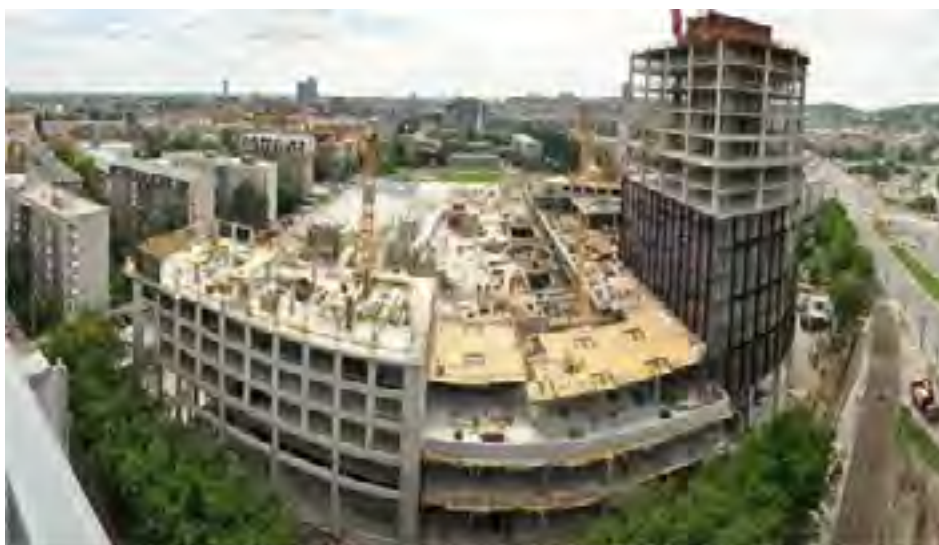
During construction time: The roof of the shopping center will offer a 6,000 m 2 natural setting and ample opportunities for an entire family to relax.
