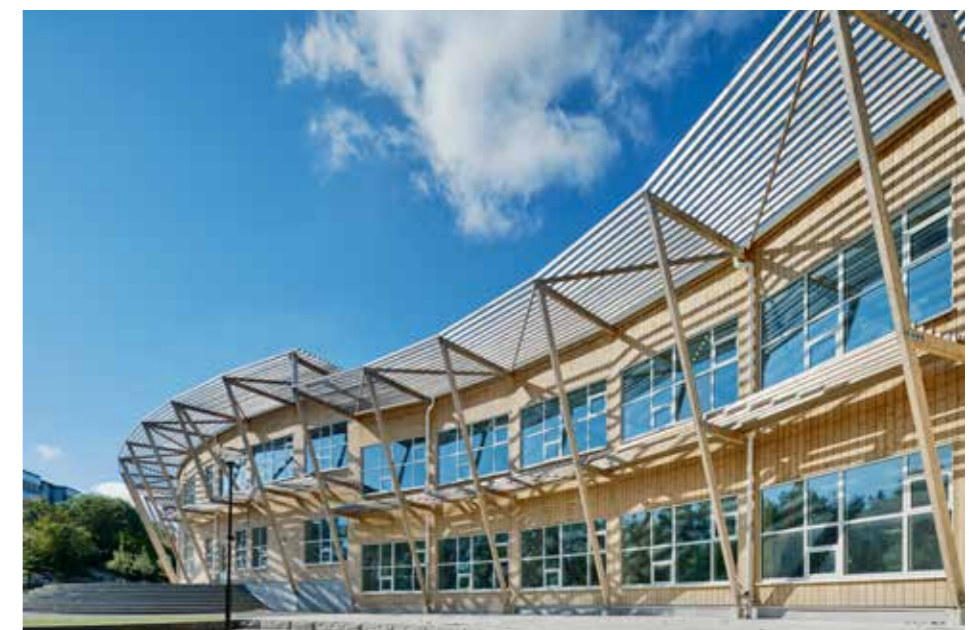
The plot is surrounded by several pine forests, which are reflected in the shape with facades of untreated or heat-treated Thermowood of pine.
