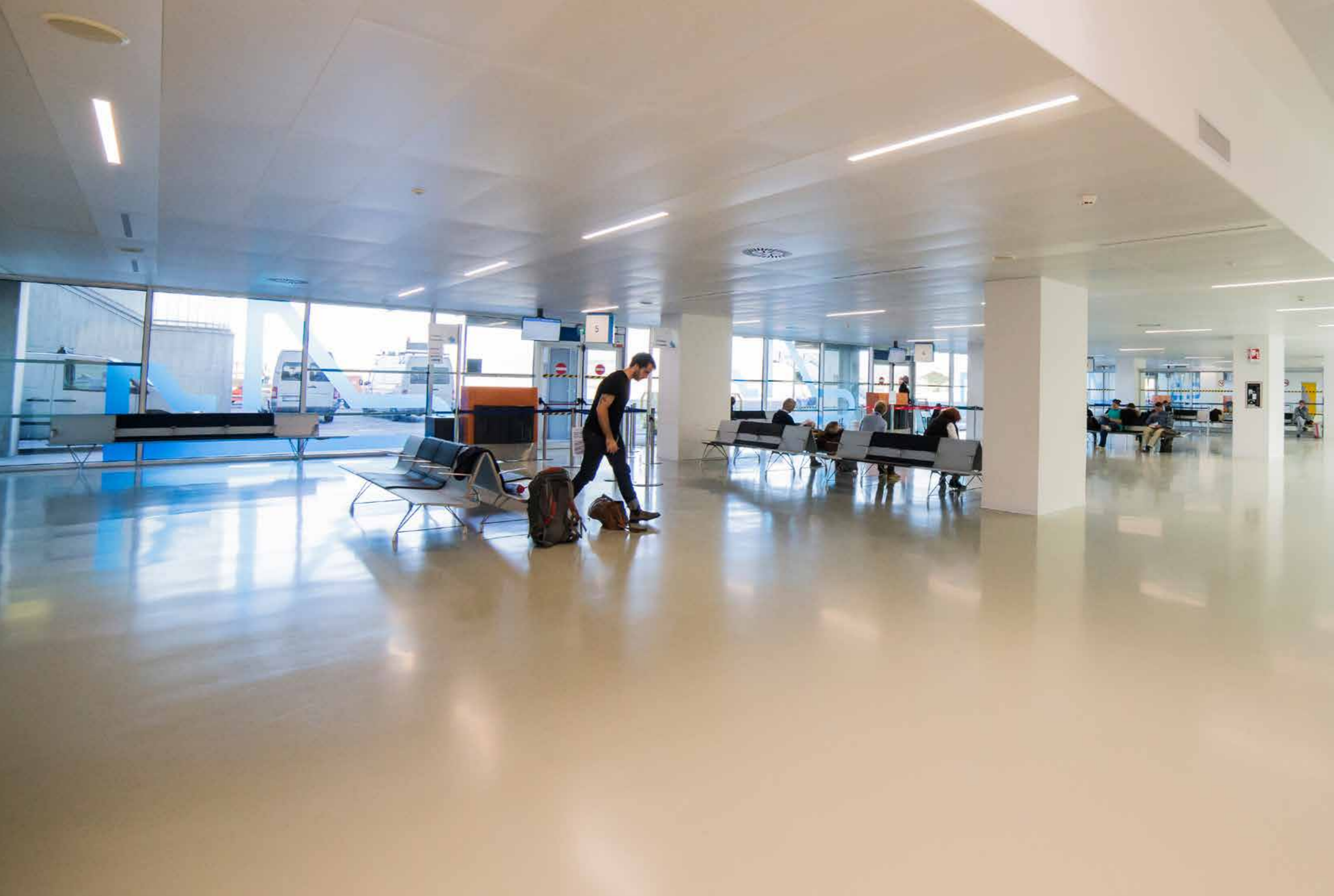
The floor has to withstand a transit volume of approx. 700,000 people per year.
