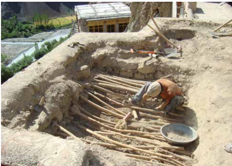
The existing roof of up to 1 m thickness was to be removed. The new roof structure is based on a double split aluminum lightweight structure.
