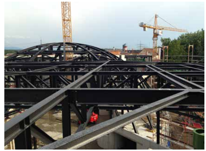
A steel framework serves as load-bearing structure for the hall and dome.
