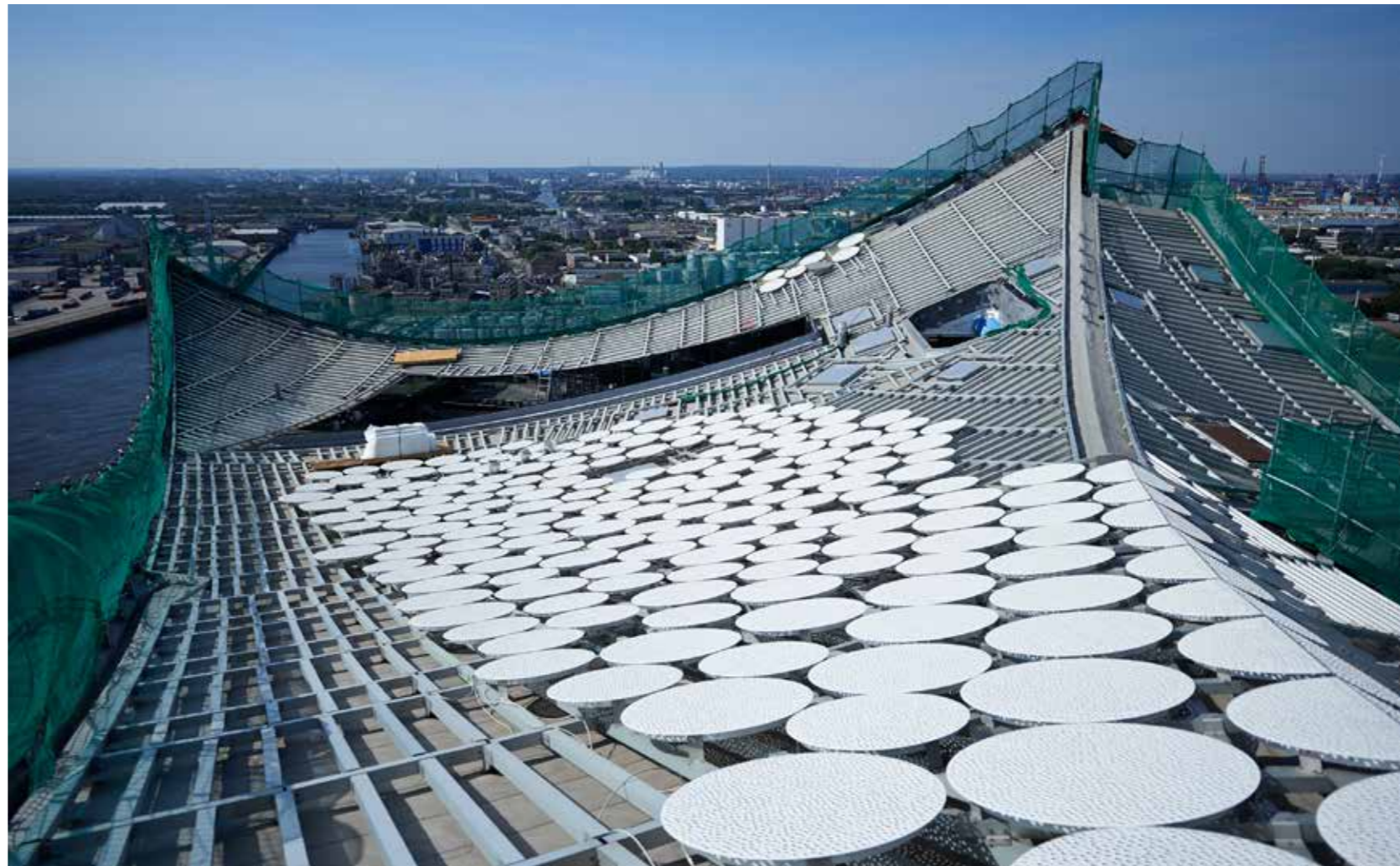
Photo to the left: Apart from the Sarnafil TS 77-20 FPO polymeric membrane, the building also incorporated other products from the Sika Sarnafil system range.
