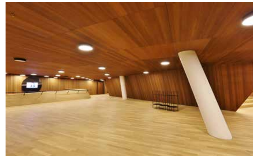
Sika sealants were also specified for the floor joints.
